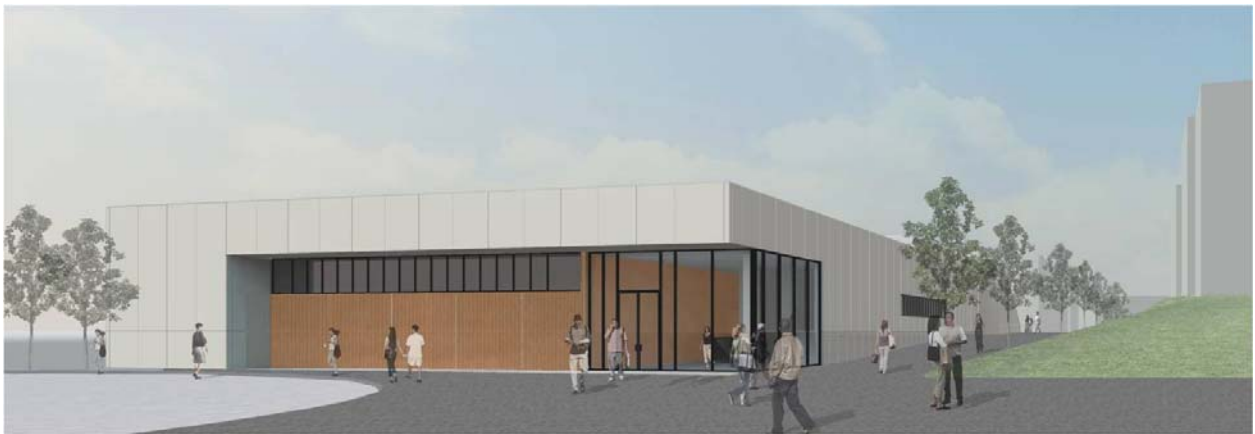
Building 4N as viewed from the drop off on the north side, looking southwest.
